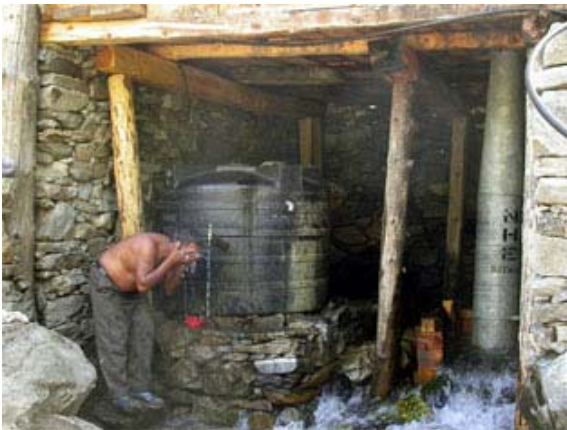
Figure 6: With 210 WLED lamps running, another 850 watts are diverted to heat water for hot showers and cooking food.
