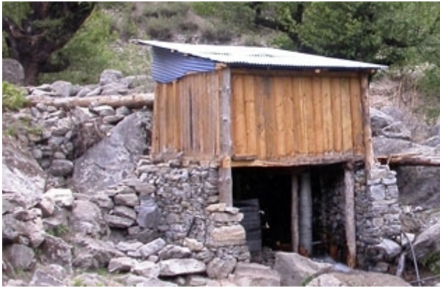
Figure 4: Beside the generator, the turbine and roof, the Pico hydro power plant infrastructure is built without any cement, using only locally available materials such as stone and wood, that creates a strong ownership among the users.
