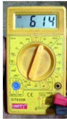
Figure 7: With 615 Volt AC the power is underground transmitted to the village.
