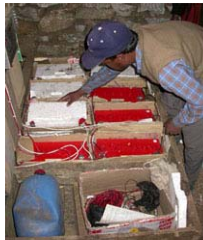
Figure 3-8: A project staff member teaches the local trainees how to check, clean and maintain the battery bank.
