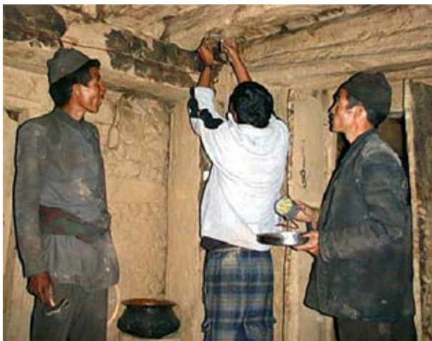
Figure 3-7: A project staff member trains the chosen local people in how to install and maintain the WLED lights, switches and house wires.
